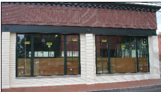
New Storefront Under Construction
